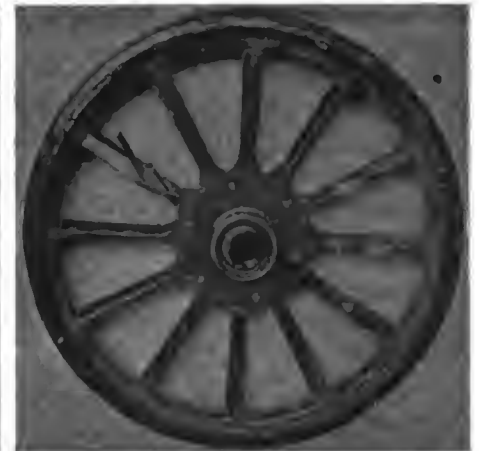
Fig. 33—Illustrating a wheel of great strength with uniform wood as selected by the Pierce wheelwright
